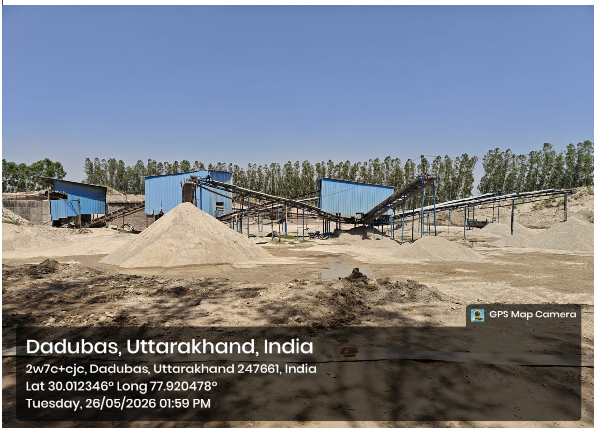
Photo: Covered shed over crushing unit and conveyor belts. Date: 26.05.2026
